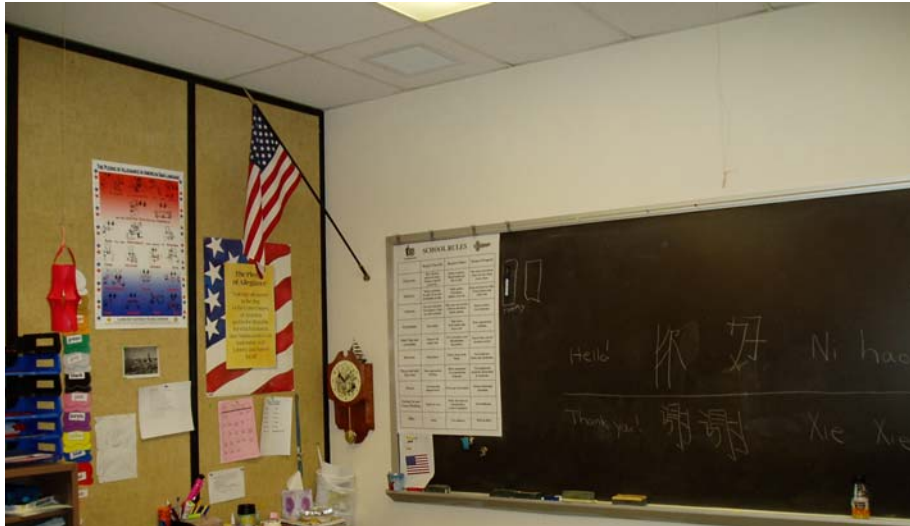
Figure 14: Photograph of classroom 5 illustrating the chalkboard covering drywall and the paneled surface (e.g. temporary wall).
