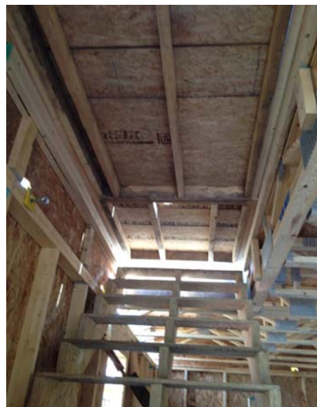
Figure 10 – Stair covers in place from below.
