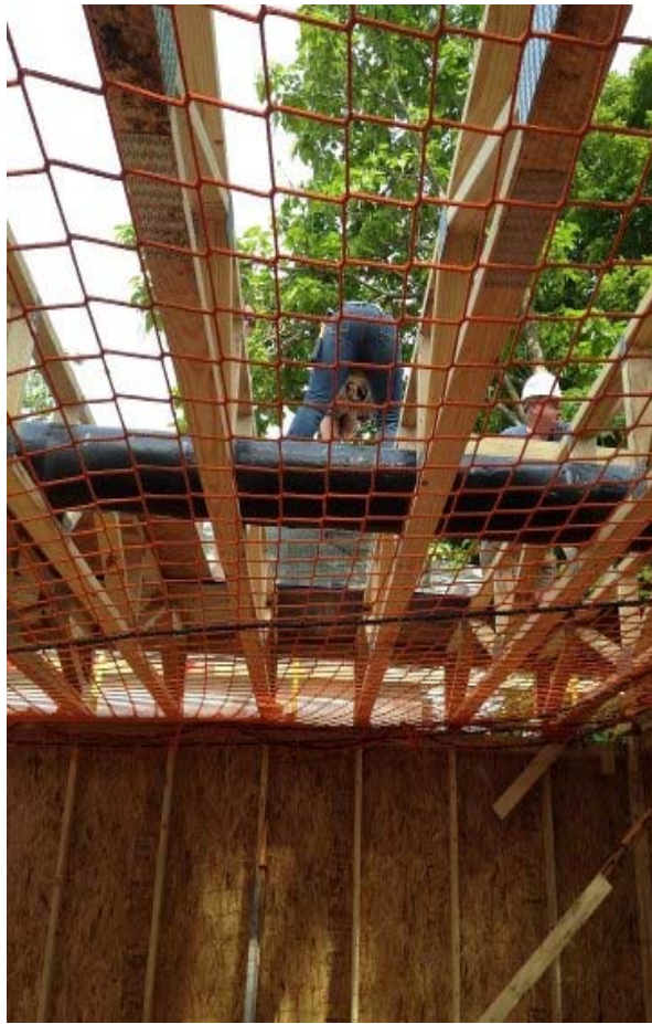
Figure 1 – Safety nets guard workers on second floor.
