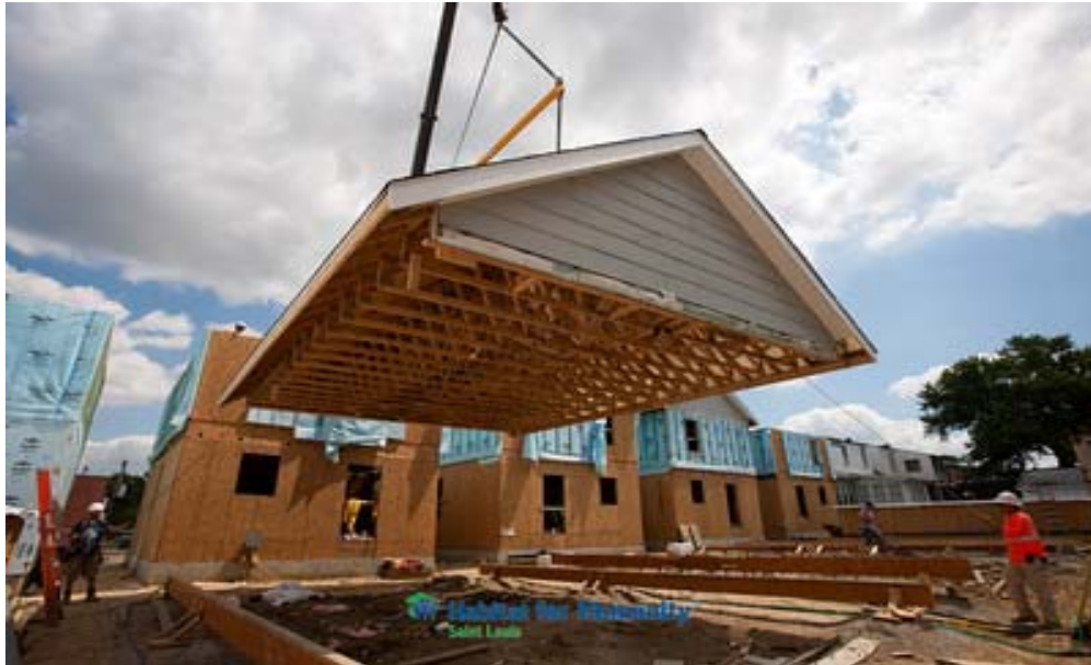
Figure 13 – Roof assembly being lifted by large spreader bar.
