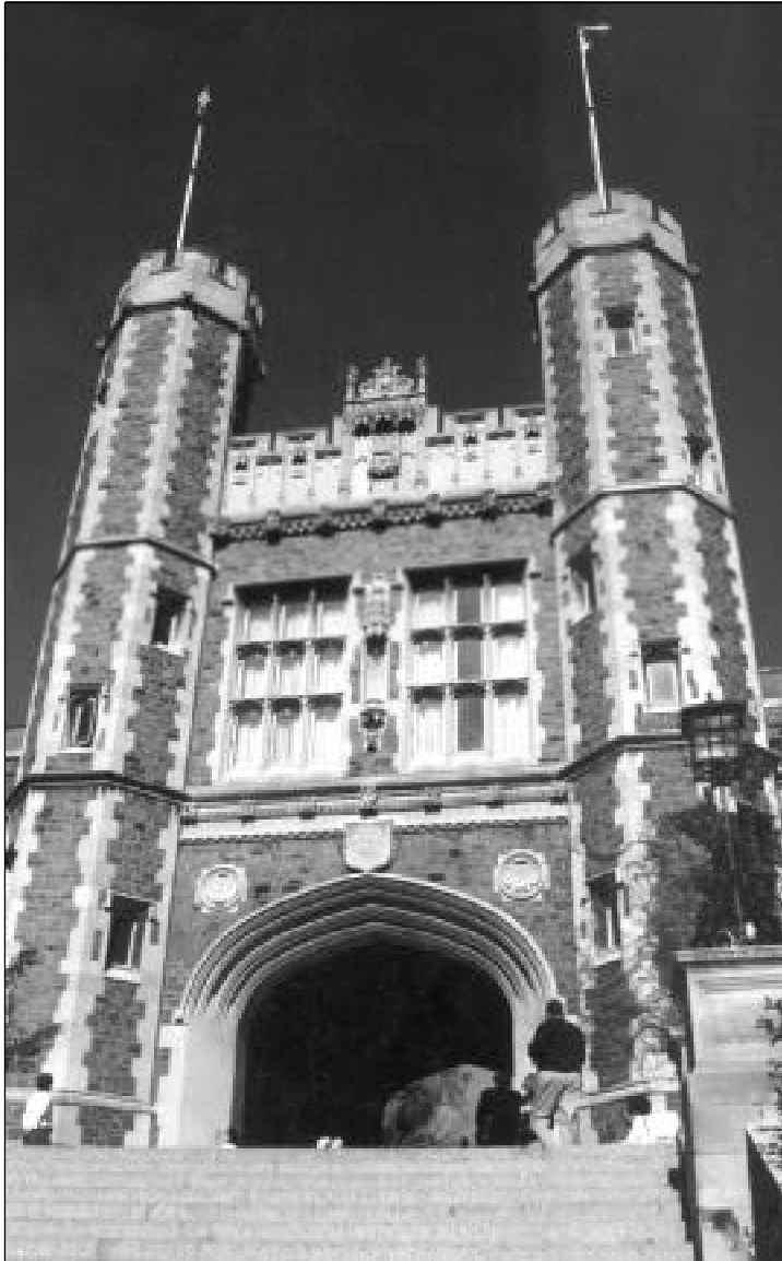
Brookings Hall, a Collegiate Gothic building reminiscent of Windsor Castle, is the hallmark of Washington University. It is the main entrance to the Hilltop Campus on the west side of Forest Park.
